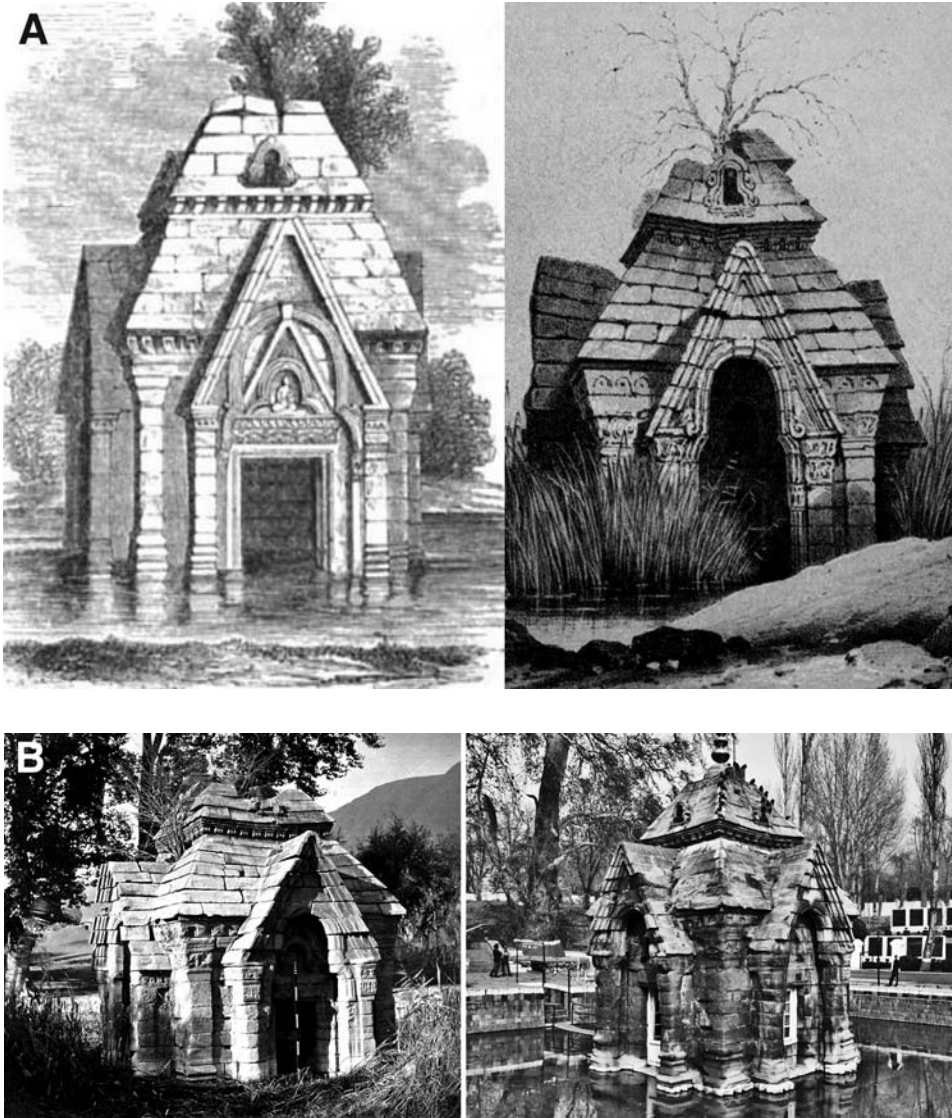
Figure 3. (A) Our earliest glimpse of Pandrethan (left) may be a sketch published by Cunningham (1848), here reproduced by Fergusson (1867), which shows a tree with abundant foliage sprouting from the roof. In the 18 July 1860 painting of Pandrethan from the north (Knight, 1863, p. 354), the internal tree is devoid of leaves (right). “The building which alone remained in at all a perfect state was situated in a sort of pond or tank of slimy green and was quite inaccessible without a boat.” He complains of mosquitoes plaguing his sketching and ants eating his paints. (B) Left: John Burke’s 1868 photo of the Pandrethan temple from the south, compared to approximately the same view in December 2008. The three upper roof courses were missing on the SE side in 1868, but are present, though dislodged on the NW side (Fig. 4). Note scale with 1 ft gradations in doorway on left.
