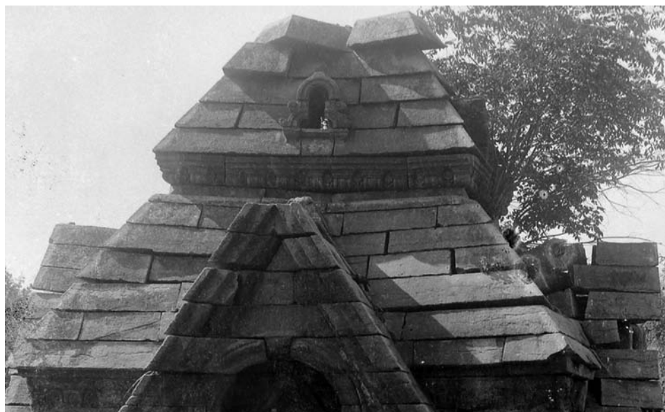
Figure 4. Close-up of Oldham's 1887 view of the temple from the NW. Note the parted SW gable (lower right) with its missing third block, also missing in Burke's 1868 photo and Kak's 1933 sketch. Note the irregular offsets to the SW of the six lower blocks, and sequentially increasing offset of the five upper blocks. The summit pyramid has been lost, and is now replaced by a modern dome with a triple-orbed pinnacle.
